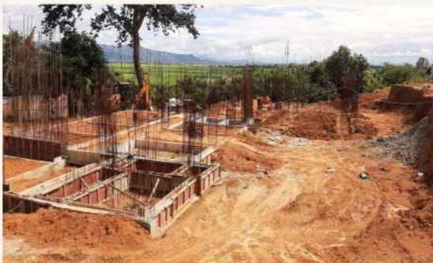
On-going construction of new campus
